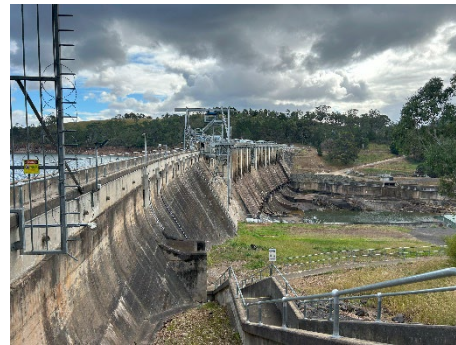
Figure 17: Glenmaggie weir dam structure.
