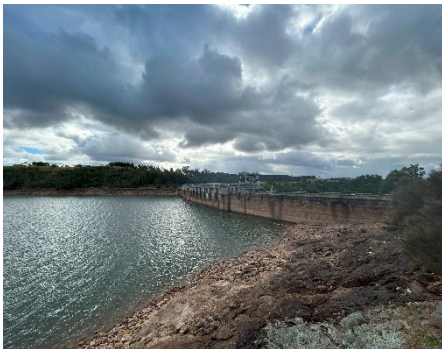
Figure 16: Water stored by the dam
